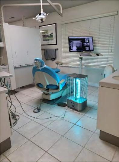
While the UV-C lamp can disinfect surfaces and the air that is passed through the lamp, it has a shadow effect. Surfaces that are not directly in the line of the UV-C light are not disinfected. Pathogens in the shadows and nook and corners are not sterilized. On the contrary, ozone, because of its permeating nature, can reach every concealed or hidden area of the room, oxidizing (killing) the pathogens.
