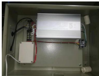
One Ballast + Relay
